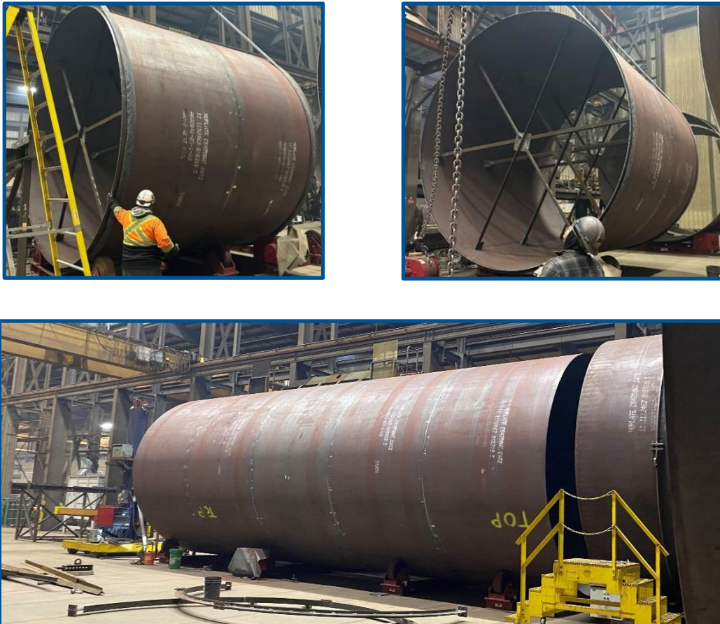
Figure 1: Typical Shop Fabrication Pictures – Cans 5 and 3
